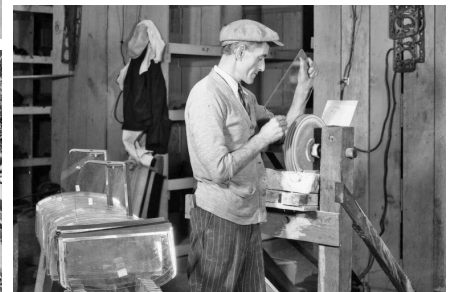
A worker grinding the edges of recycled glass into panes used for replacement wind-wings visible on the left. Note the crude shop-made glass grinder with adjustable wooden shaft bearings.
