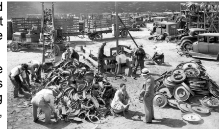
Two views (above and below) of the metal shear used to reduce wheels and other components into pieces. Note the conveyor belt used for loading scrap into trucks and trailers.
